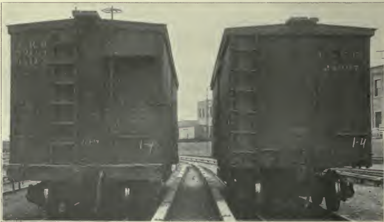
FIG. 512. YARD TRACK CONSTRUCTION, 600-VOLT OVER RUNNING THIRD RAIL Position of Freight Cars with Reference to Third Rail, Sunnyside Yard, Pennsylvania Railroad, Long Island City, N. Y.
